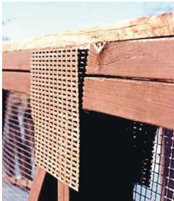
There are many ways the plate corrosion shown could have been avoided.
