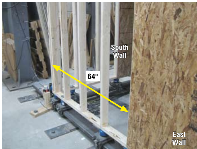
Photo 5. Due to the 16" typical wall panel stud spacing available to SBCRI at the time of this test, the first 3/8" OSB braced wall panel was installed 64" from the south end of the wall. The OSB panel on the north end of this braced wall line was set 72" from the end of the wall.
