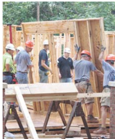
Volunteers set the walls mid-day on Day 1.
