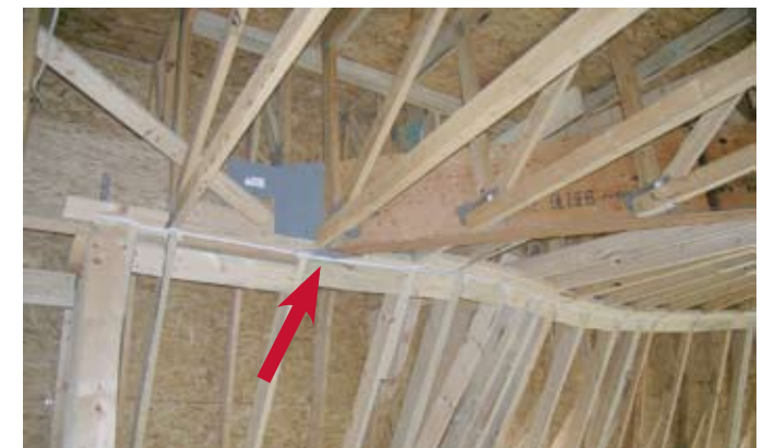
A cantilevered beam (top left) carries the beam that runs across tower at a 45 degree angle (top right). An identical configuration is replicated on the opposite side. “The two cantilevered beams are one-piece param to avoid concerns over the hanger distributing load to multiple plies in a very short cantilever,” Heinsman said. Kolosky and Heinsman worked together to adjust the placement of the beam to allow the scissor trusses to tie into it and simplify the installation.
