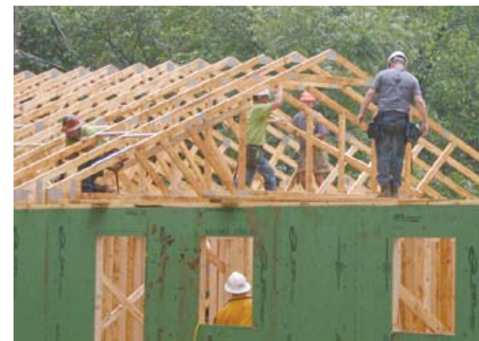
The roof trusses were set Day 1.
