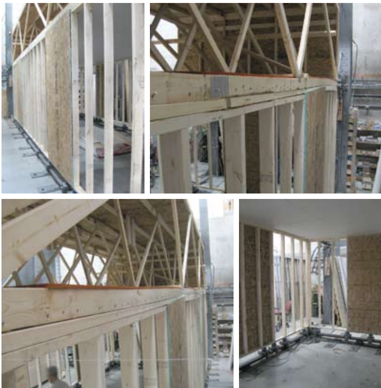
Views of the 12'x30' IRC-compliant structure in SBCRI. Braced wall panels are placed in various locations along the structure, loads are applied, and the products' performance is measured.
