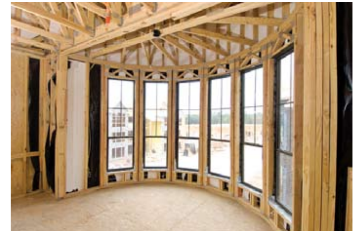
Harris says like traditional wall, roof and floor components, its plated headers, corners and other rough openings offer builders and framers tremendous value in many areas.
