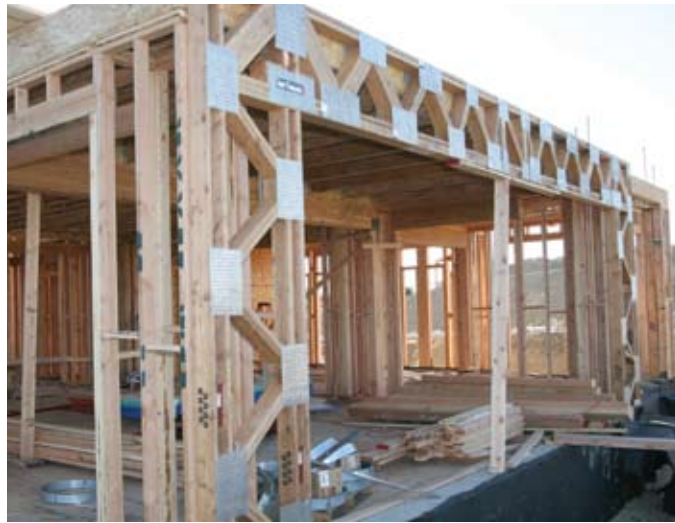
A "Smart Portal" installed in a California residence. Turning more of the house into components is the key to regaining market share, says Cloyd.
