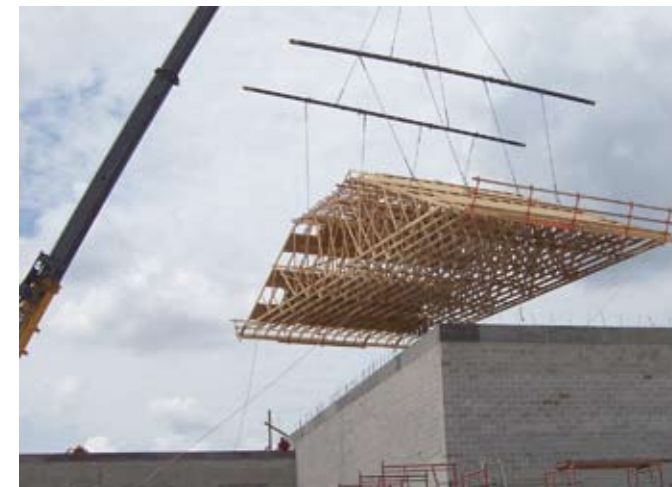
Sheathing and bracing was applied before hoisting this assembly of more than 20 trusses.
