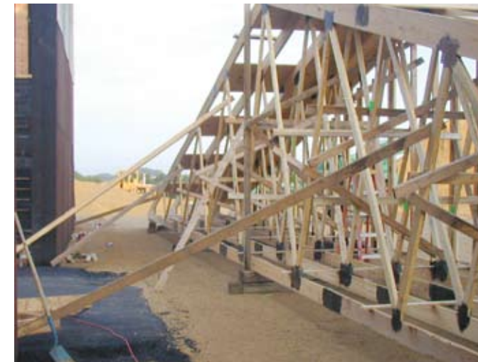
Ground Bracing for truss assembly being built on the ground.
