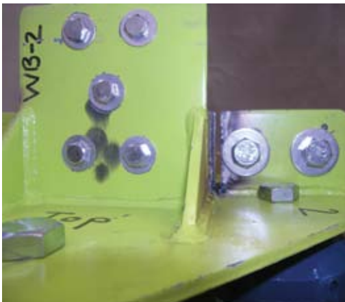
Figure 5. Close-up of the top plate of WB2.
