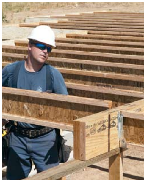
Precision-cut and labeled floor members benefit builders by reducing construction cycle time, call-backs and jobsite waste, while improving quality.
