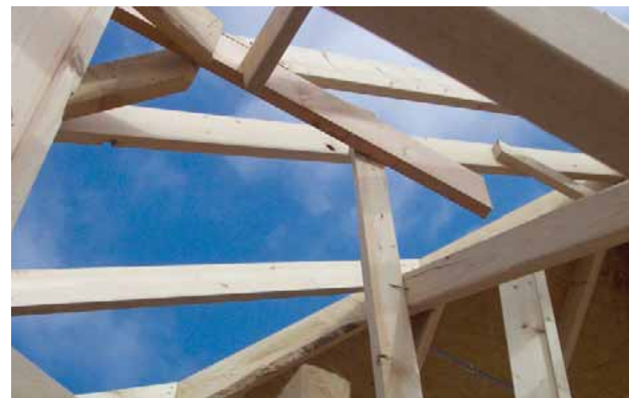
The end of a ridge beam for a dormer is bearing on a 2x4.
