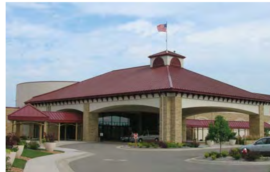
For this casino expansion project, converting cold-formed steel trusses was a "no-brainer."
