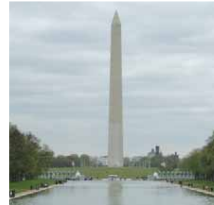
Photo courtesy of Jim Swain, Carpenter Contractors of America, Inc.
