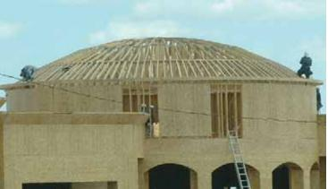
This recently completed retail building in Las Vegas, NV features bow-string trusses. Justin Henricksen, a truss technician in the Las Vegas area, designed the trusses for the domed structure. Henricksen says he has been seeing quite a few requests for the bow-string trusses, although this one was their biggest so far at 58'. He commented, "Everybody wants to do these round towers, it seems to be the norm right now."
