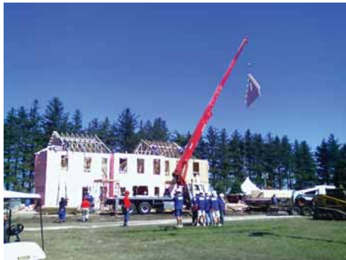
A roof truss is hoisted into place on the Cascade site.
