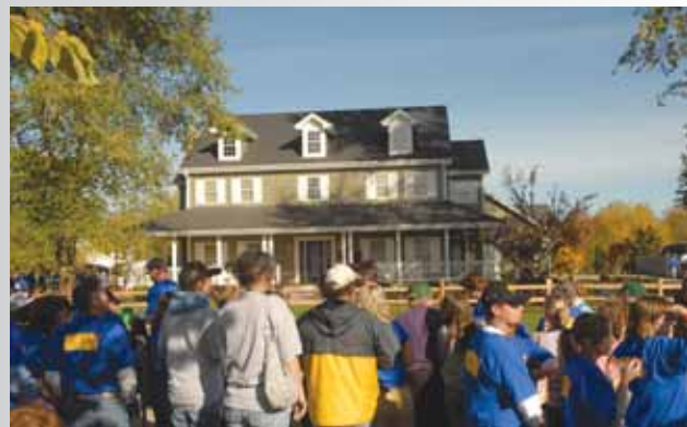
In just one week, 1,500 volunteers pulled together to build this 3,740 square foot country colonial home with a wrap-around porch with dormers for the Koepke family of Dundee, WI.
