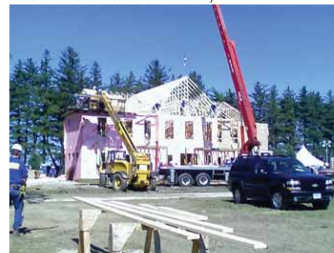
The Cascade house as it was starting to come together.
