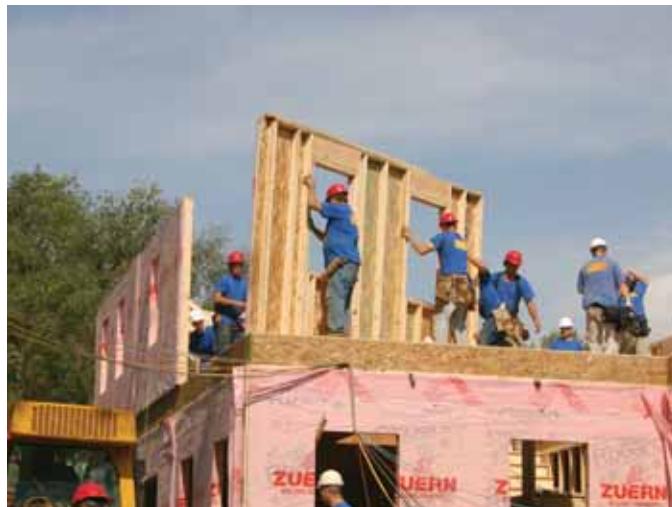
Framers set wall panels in place on the Richco site.
