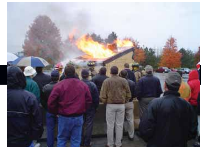
At 13 minutes, 11 seconds. The concentrated loads bearing on the sheathing have now fallen through. One point made by the demonstration is that sheathing typically fails in fire before the structural members.
