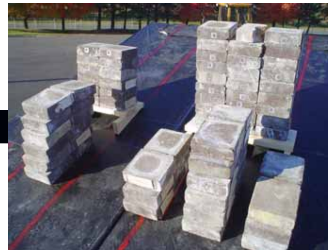
The concentrated live loads were applied using 22-lb. bricks. The joists on the left carried 528 lbs, and the trusses on the right carried 1112 lbs. The joists and trusses were equivalently stressed under these loads. See www.fire.carbeck.org for a more detailed description of the demonstration design.
