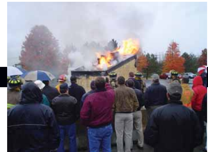
At 12 minutes, 15 seconds, the fire penetrating the floor indicated significant gaps in the decking on the truss side. At 12 minutes, 51 seconds, both the joists and the trusses are still holding load.
