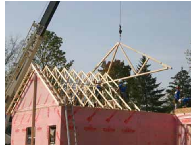
Roof trusses for the garage being set on the Richco site.
