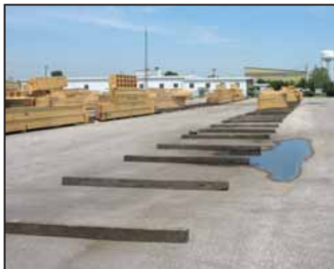
Trusses or truss bundles stored flat on the ground should be raised a few inches by blocking at 8' to 10' on center.
