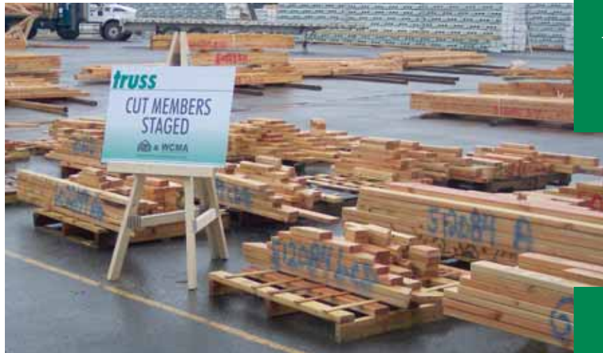
A cold mist falls on the cut members staging area in the BMC West yard.
