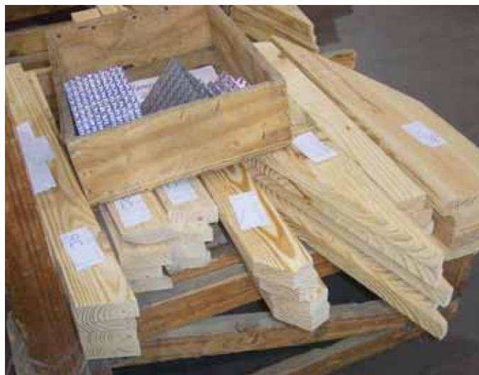
A box on top of cut webs contains the precise number of connector plates for that specific truss.
