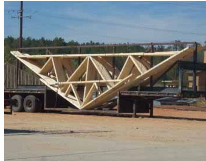
Roof trusses are stacked vertically on a custom-built trailer.
