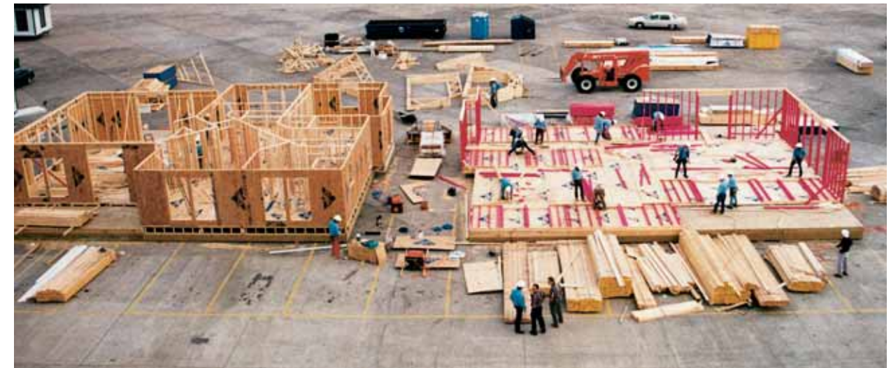
The 1996 Framing the American Dream® project helped to illustrate the many benefits of building with wall panels (see list on page 8).
