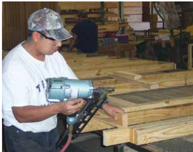
Wall panel line worker prepares to nail header.
