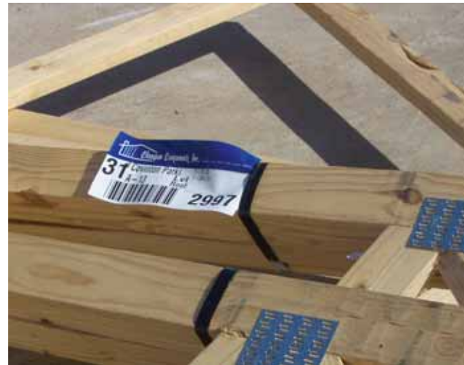
Banded trusses are tagged with the job title and number, truss type and number (for placement during framing). The bar code is scanned by a dispatcher as the trusses are loaded for delivery.
