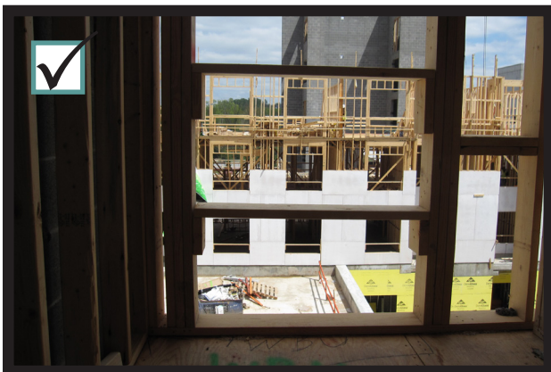
Erect guardrails around window and door openings.
