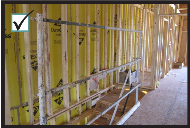
Erect guardrails around stairs.
