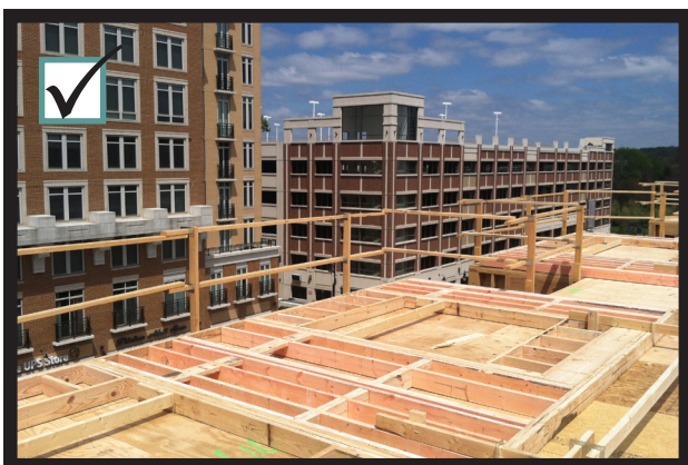
Erect guardrails around the leading edge.
