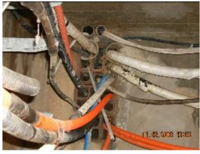
The Baltimore City Conduit system consists of pipes or "ducts" used to protect and route wiring underground in the City's Right of Way (ROW). The ducts are made of either plastic, fiber, or Terra Cotta. Conduit is installed underground between multiple manholes, buildings, structures, or devices to allow for power and communication cables to connect buildings, businesses, and homes.<sup>28</sup>
