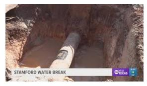
This damage occurred November 4, 2025 when a Syntrio construction crew bored through a 16-inch water main — the largest in Stamford, Texas — while installing underground fiber lines. The crew called for utility marking but started digging within 20 minutes of making the call.<sup>27</sup>
