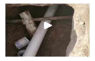
Without careful planning, bad results such as this one can happen, where Spectrum ran their fiber optic cable through a homeowner's sewage line, not only destroying the line but also allowing city sewage to backflow into their home, costing them \$20,000 in damages.<sup>26</sup>
