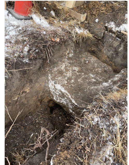
Excavation uncovered remnants of old concrete below grade.
