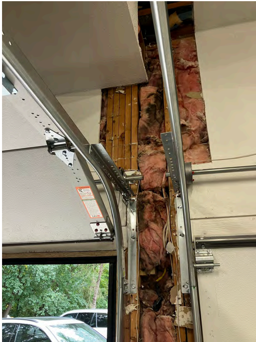
Old support configuration over garage.
