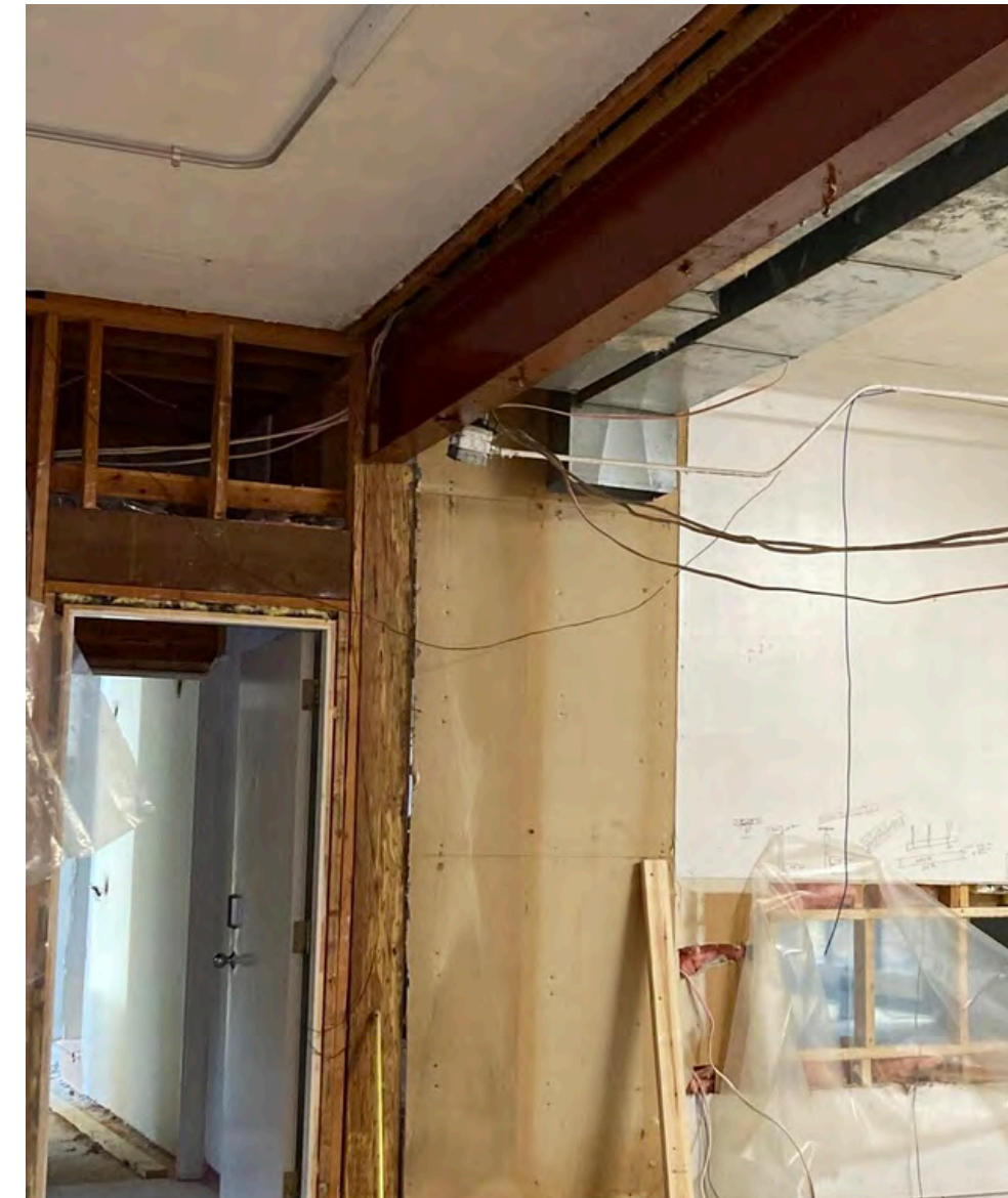
New support installation leading into mudroom.
