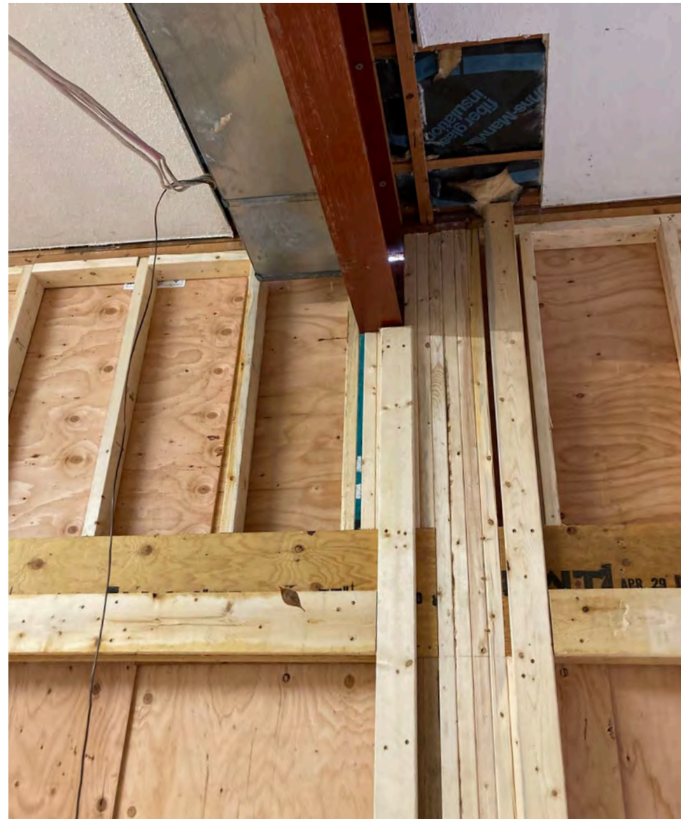
New support installation over garage.
