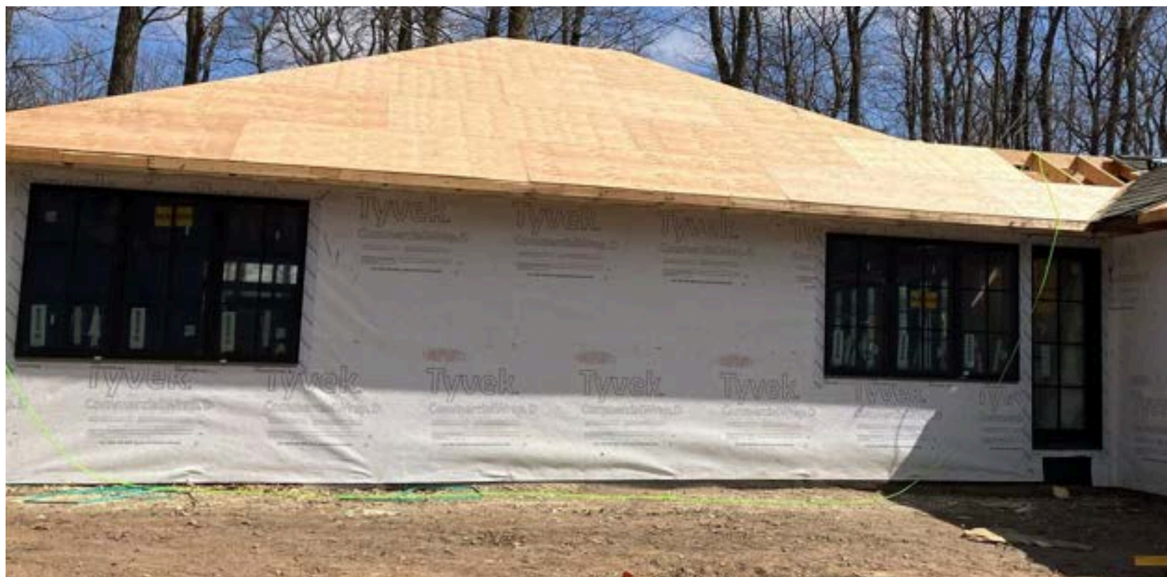
Ready for roofing
