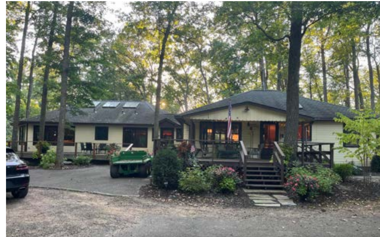
Original structure and 1980s addition
