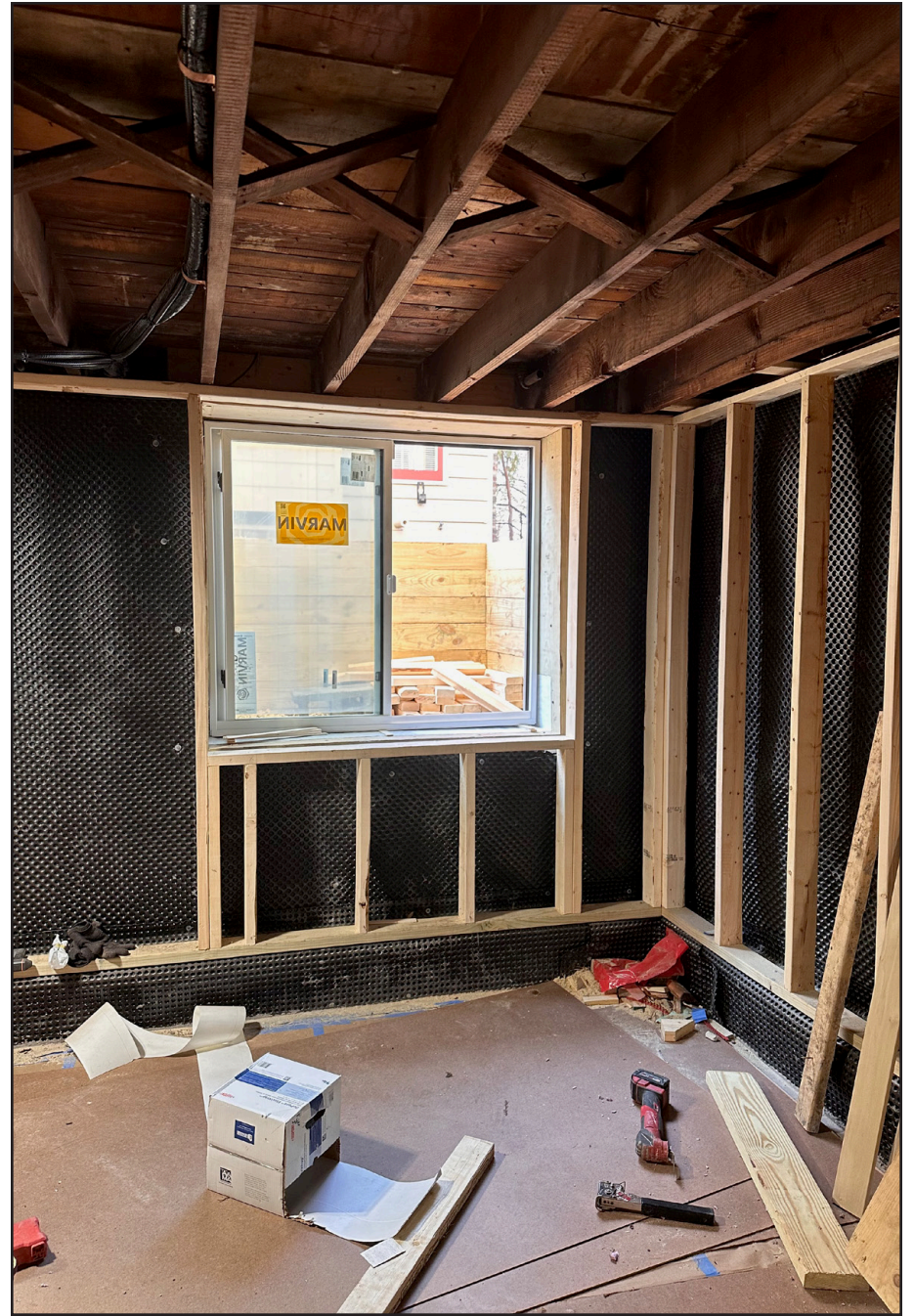
New underground plumbing and drainage were installed for the reconfigured bathroom, laundry and mechanical systems. Enlarged window openings improved daylight and egress, while perimeter waterproofing and new framed walls strengthened the basement envelope.
