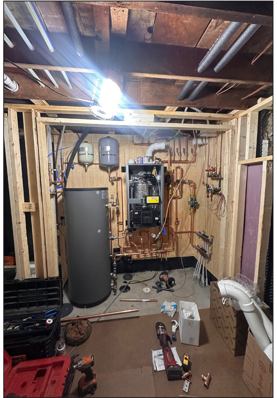
Rigid insulation was installed beneath the new slab, with radiant tubing above it to create a warm finished floor without sacrificing headroom. New high-efficiency mechanical systems were consolidated into a compact utility zone, freeing valuable floor area elsewhere.
