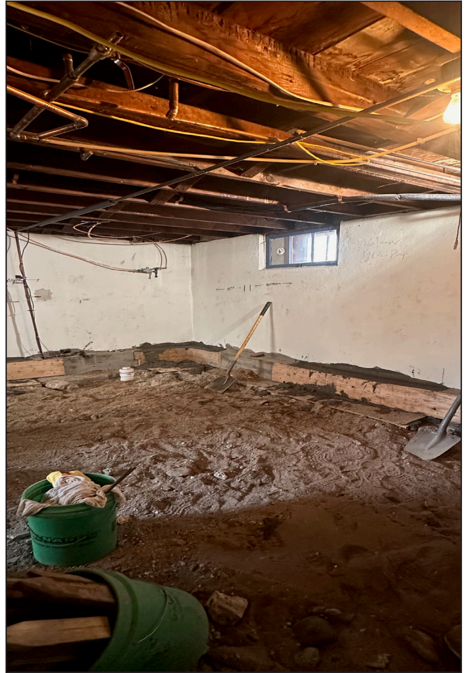
The original foundation walls had no footings, requiring new footings to be incorporated as the basement was excavated for additional headroom. The walls were underpinned in four foot long sections, allowing the floor to be lowered while maintaining the existing masonry structure.
