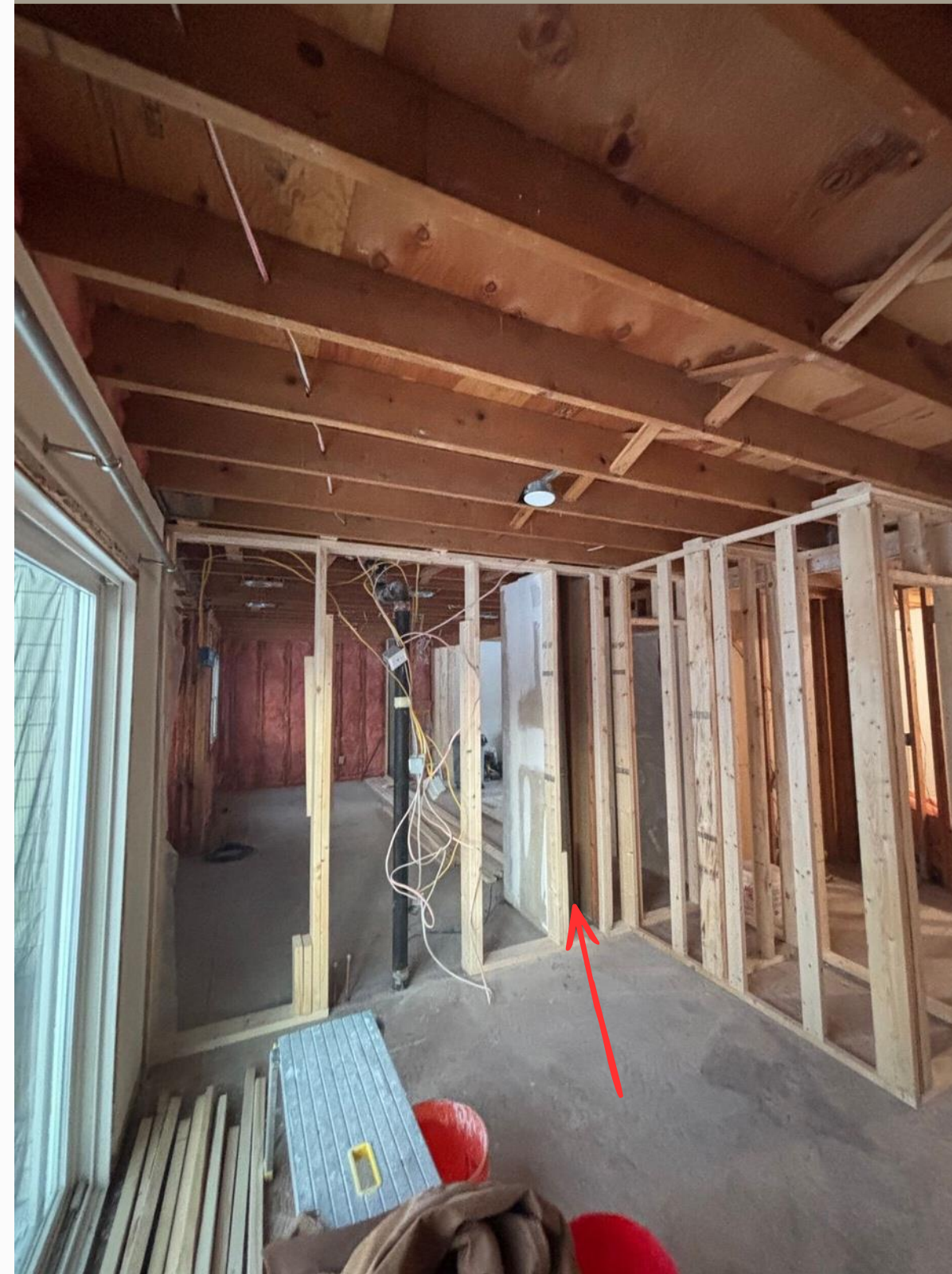
Just before beam installation
