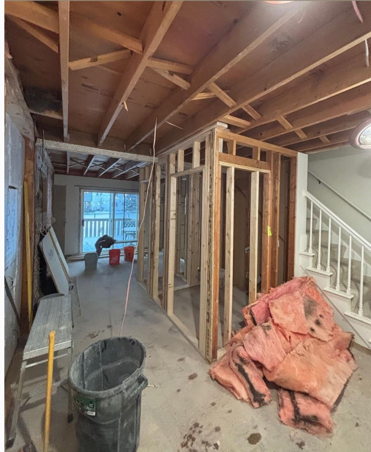
Framing in the new bathroom and extra closet storage.
