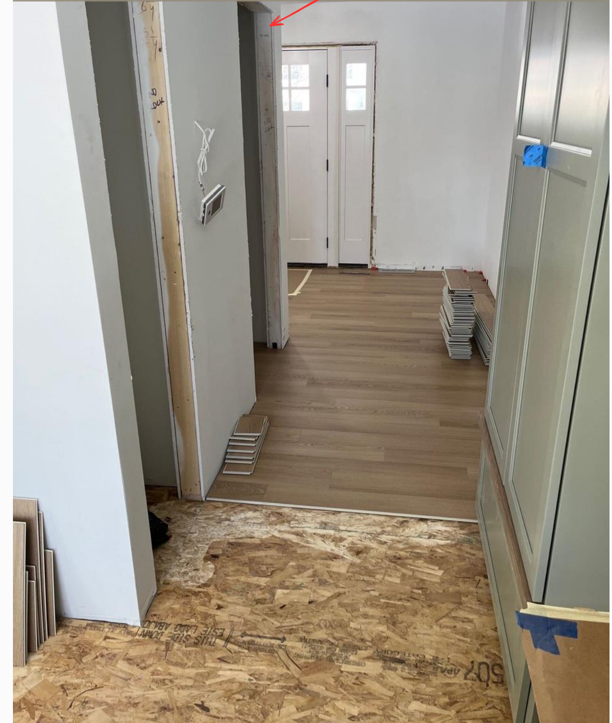
Easy access to the new bathroom from the front entry and garage.
