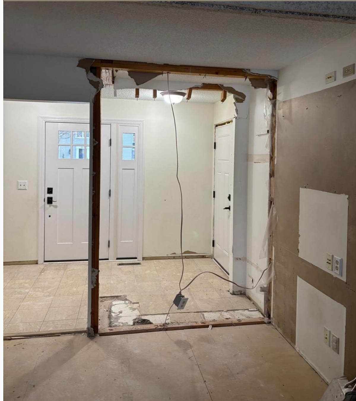
Removing the old coat closet allowed for a new walkway and extra space for the new powder room.
