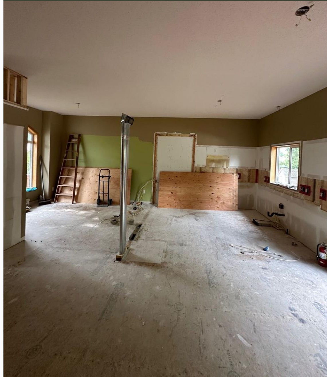
Finding solutions for the HVAC lines and framing the closet to go to the ceiling (left side of photo)
