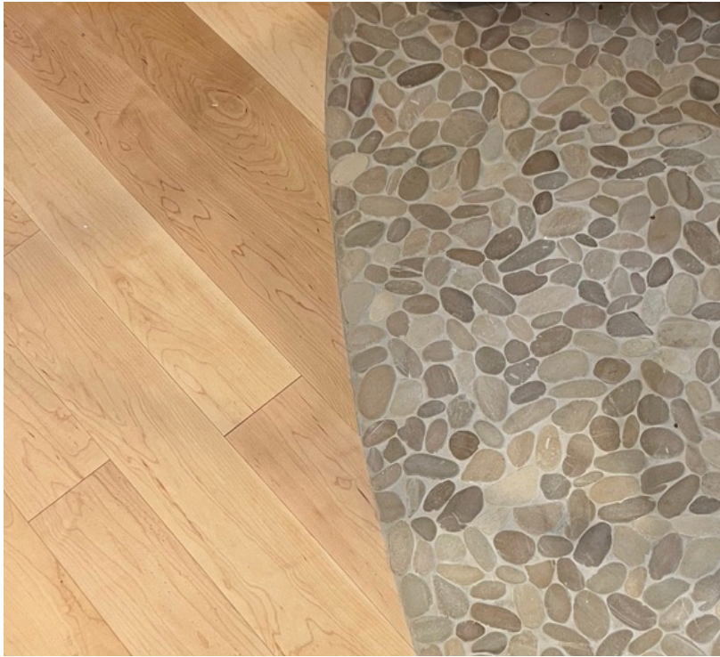
Pebble tile installed with thoughtful placement along a curved edge.
