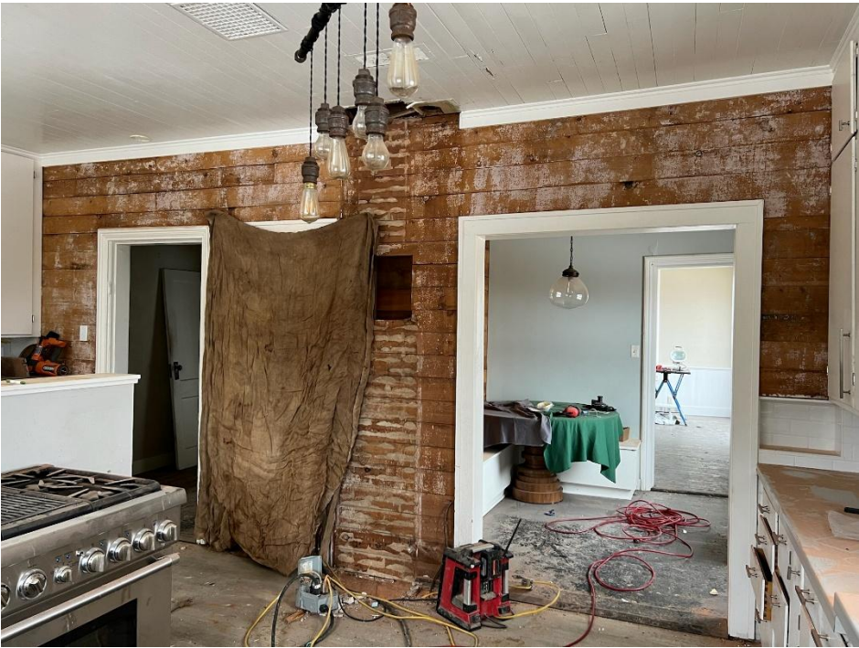
EXISTING KITCHEN (ORIGINAL WOOD WALL)
