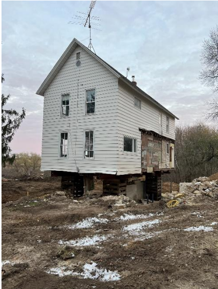
FARMHOUSE WAS PULLED OFF IT'S FOUNDATION AND MOVED 12' EAST & 6' NORTH
