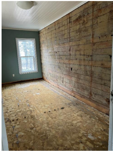
BEFORE - SMALL GUEST BEDROOM NOTE: EXISTING WOOD PANELING BEHIND SHEETROCK
