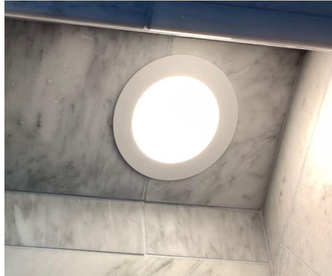
Recessed lighting is tucked in the angles on the shower ceiling.
