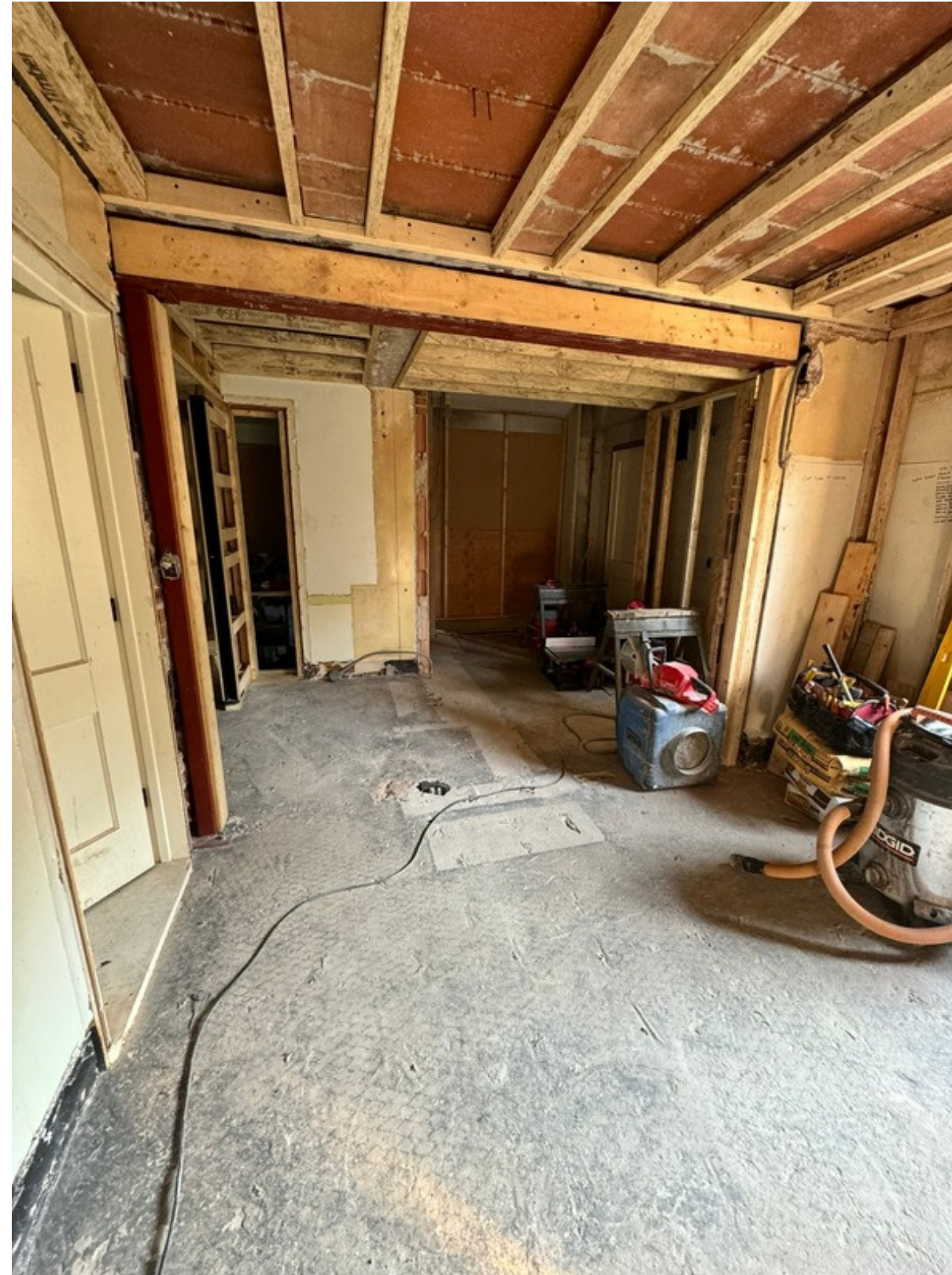
Photo showing the clay tile construction
