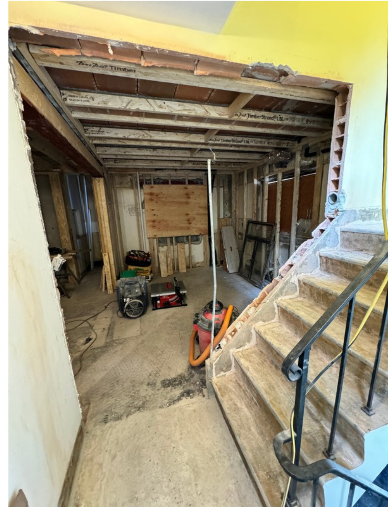
Photo showing the concrete floor, concrete block and demolition of stairway wall
