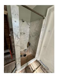
The plan was to keep the marble slabs undisturbed, but a liner was required for waterproofing the new shower pan.
