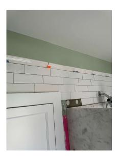
To prevent water damage the chair rail and wainscot were taken up and around the marble slabs to encase the showerhead.
