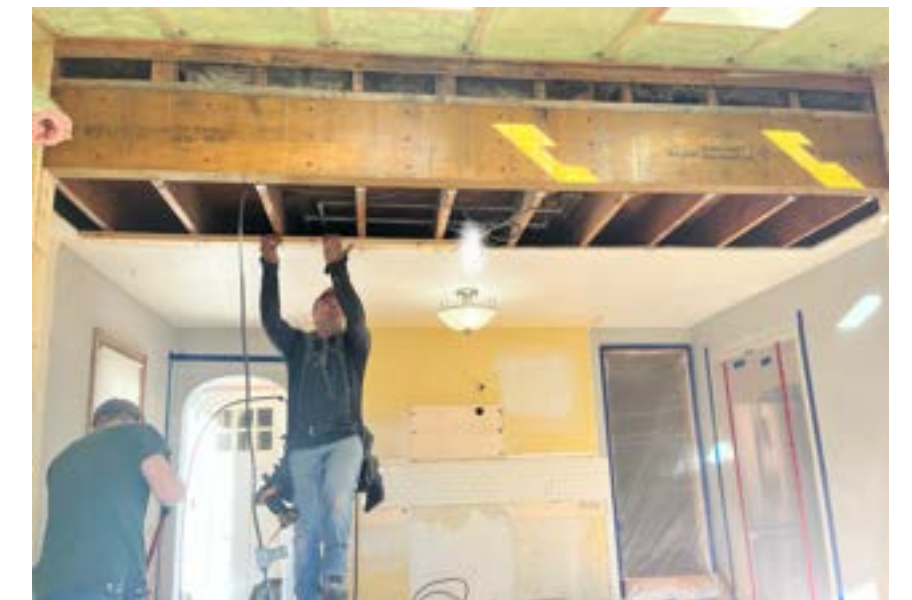
BEAM INSTALLATION
