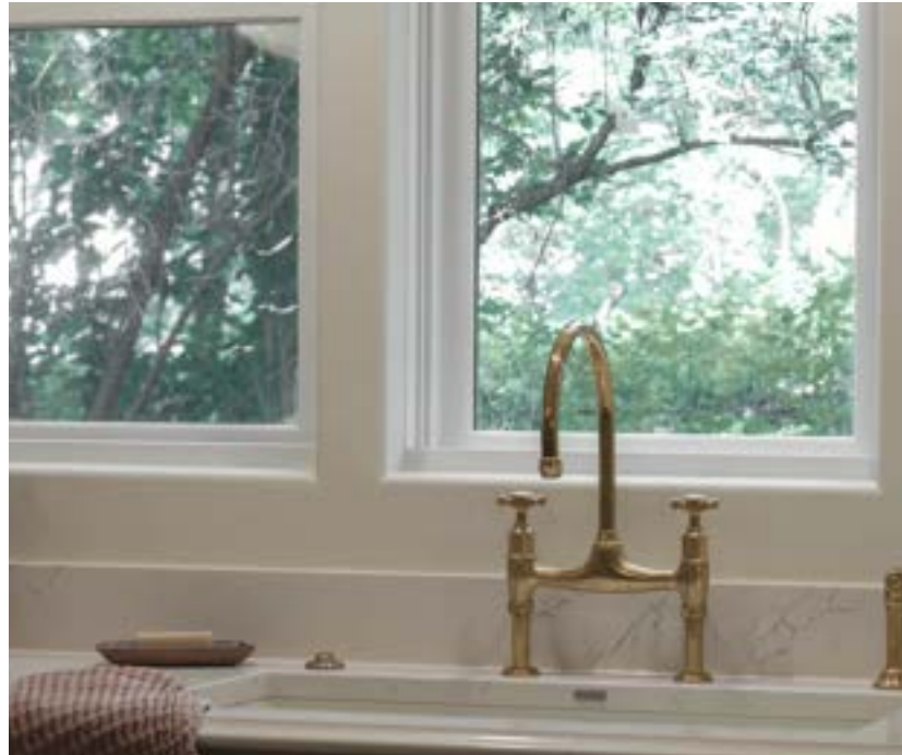
Bullnose window jambs introduce a sense of softness into the space
