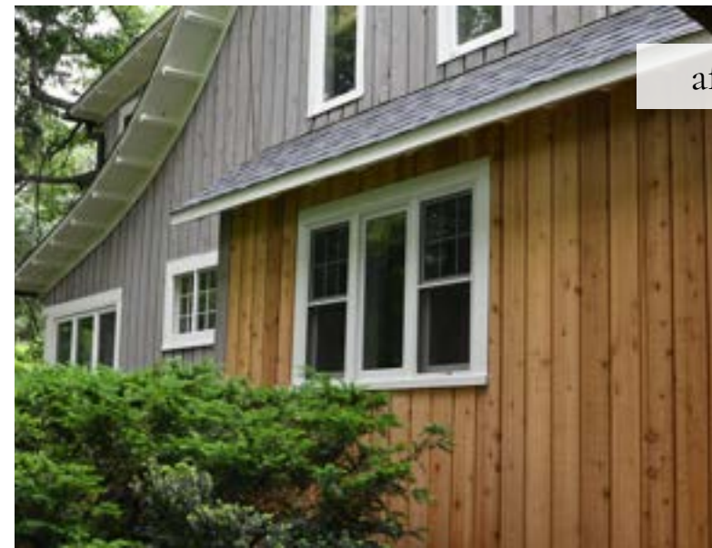
Bump out floor framing
