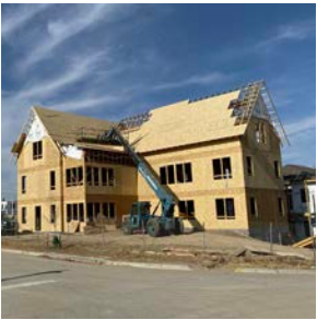
Figure 2.4 The simple forms, smaller size, and compatibility with simple wood-frame construction help maximize affordability and investment returns, and are consistent with the construction strategies familiar to most residential homebuilders, as shown in this under-construction MMH project in Papillion, Nebraska.
