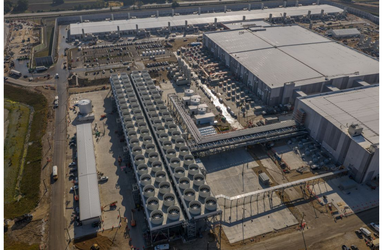
Aerial view of Microsoft's new AI datacenter campus in Mt. Pleasant, Wisconsin (September 2025).
