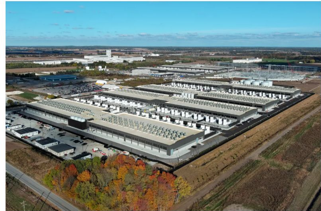
Project Rainier, an $11 billion Amazon AI data center, on Thursday, Oct. 30, 2025, between New Carlisle and South Bend.
