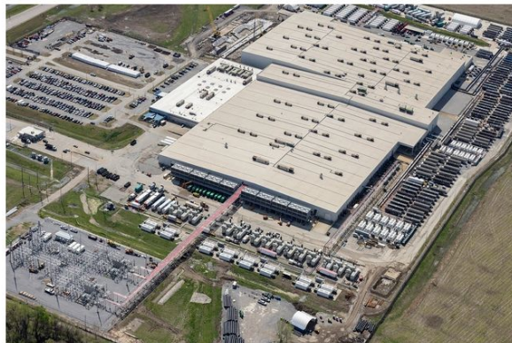
An aerial view of the xAI data center. | Steve Jones/Flight by Southwings for SELC
