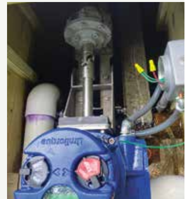
Limatorque electronic motor that operates Slide Gate 2 and controls flow coming into the mill.
