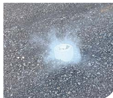
Smoke testing on a broken clean out.
