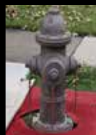
PREPPED FOR PAINTING
