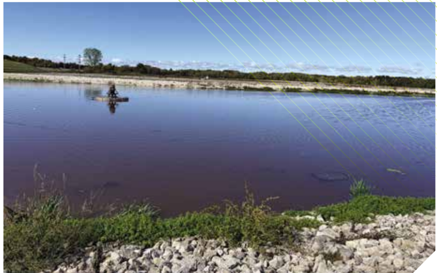
Image 3: Photo of pond on October 7, 2025 following decant of approx. 1MG of supernatant. Post ProO2 operation. (Simpson, R. 2025)
