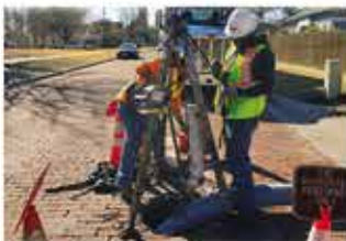
CURED-IN-PLACE PIPE
