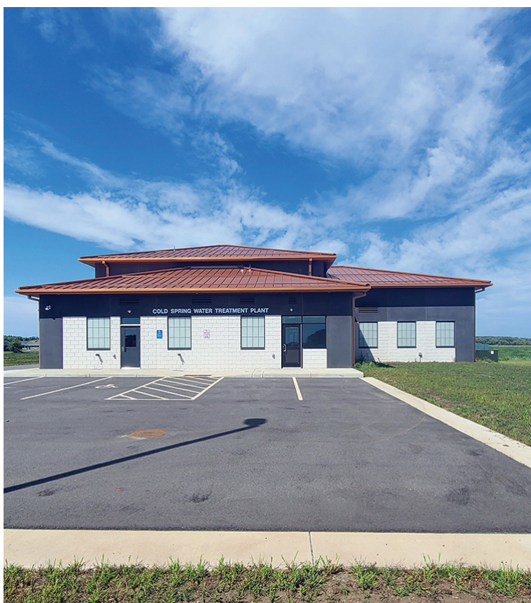
The exterior of the new plant.
