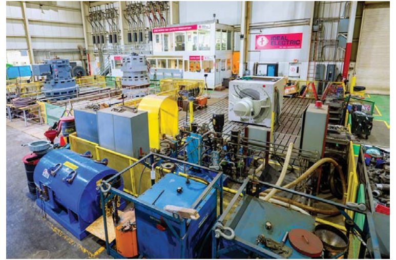
The Ideal Electric Company tests electrical equipment at its Mansfield, Ohio facility.
