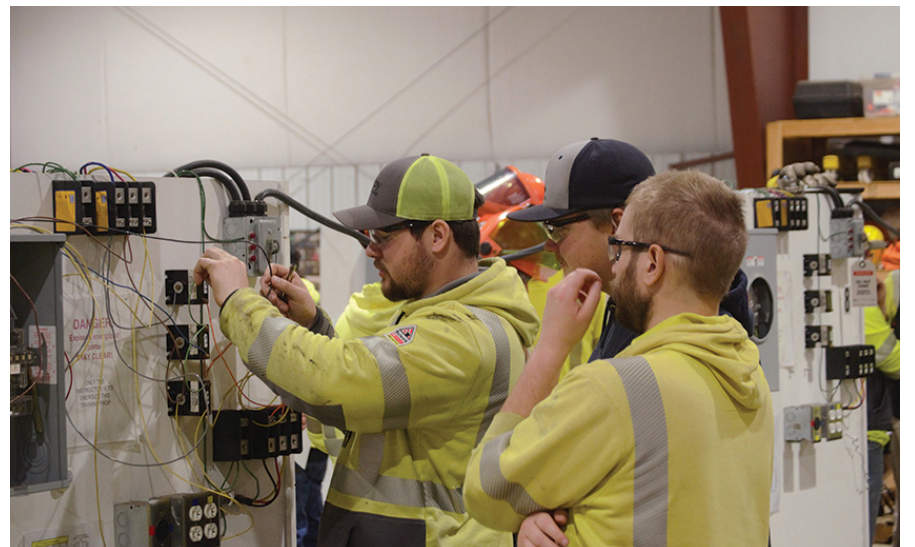
Attendees made sure the wiring was exactly right.
