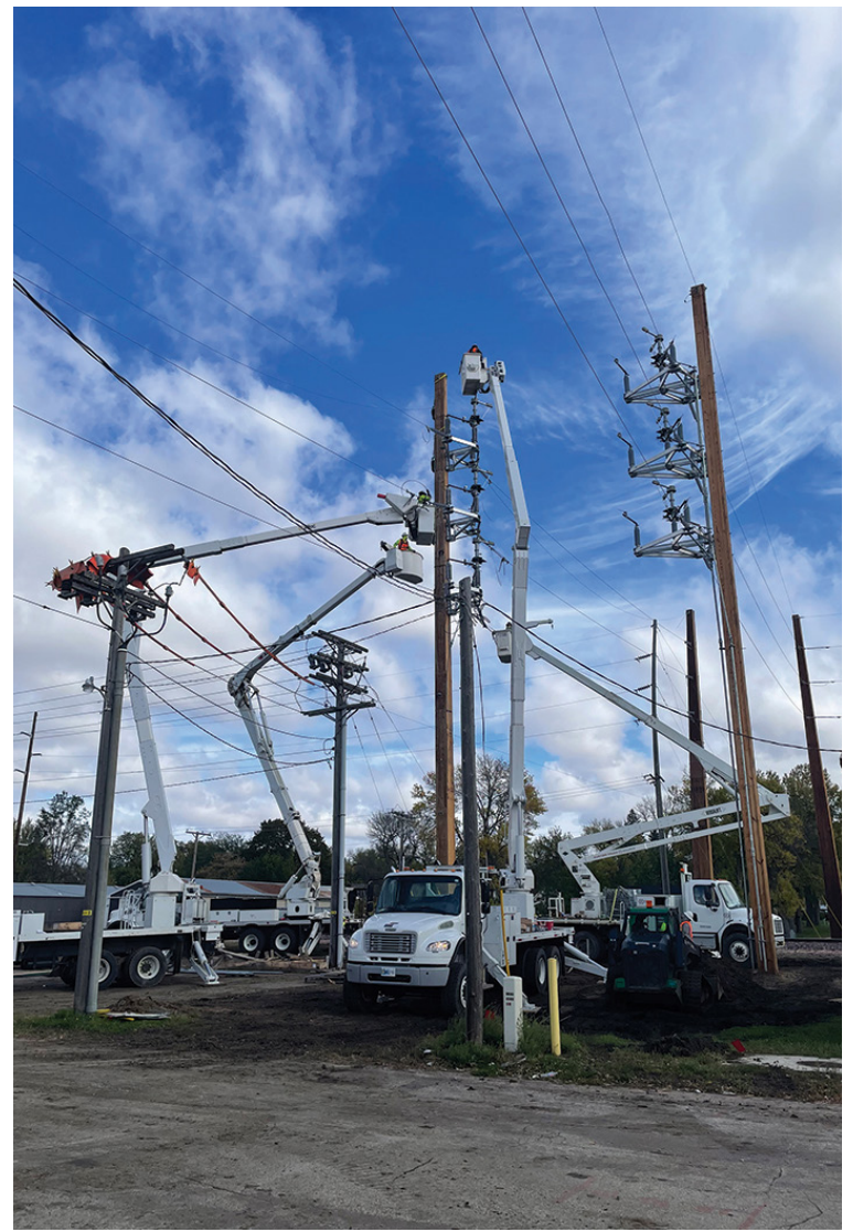
Working on the new transmission switch right outside the substation.
