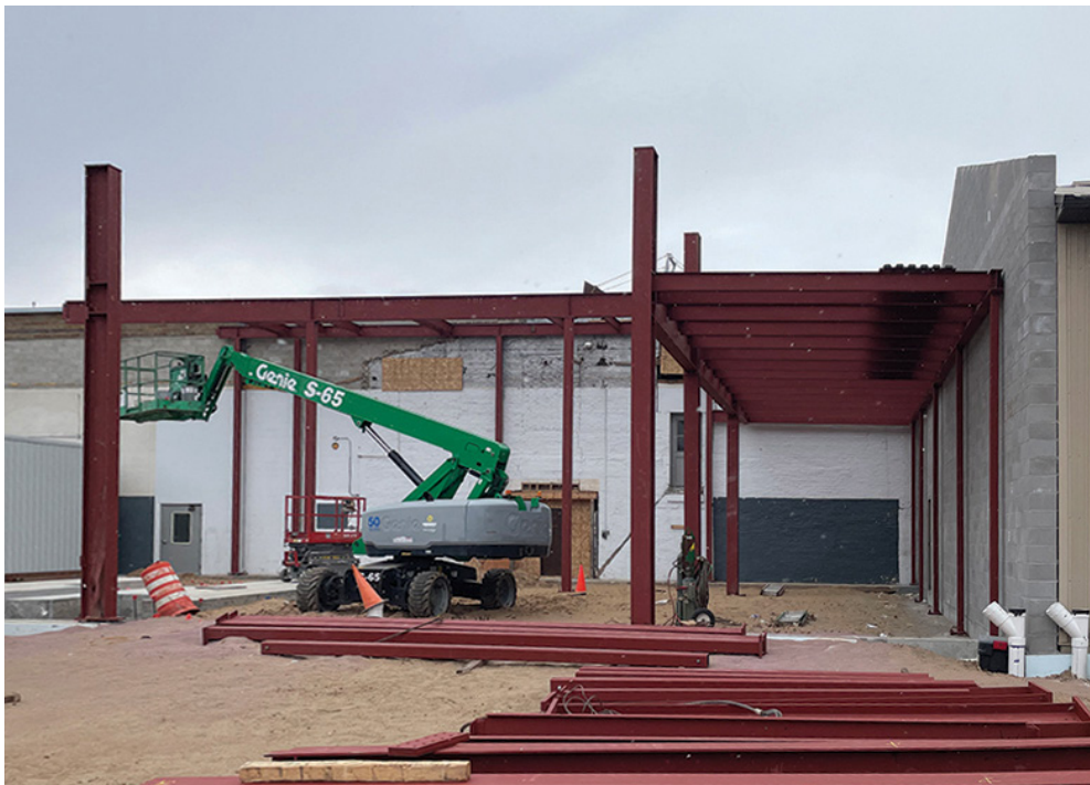
The new generation plant structure under construction.
