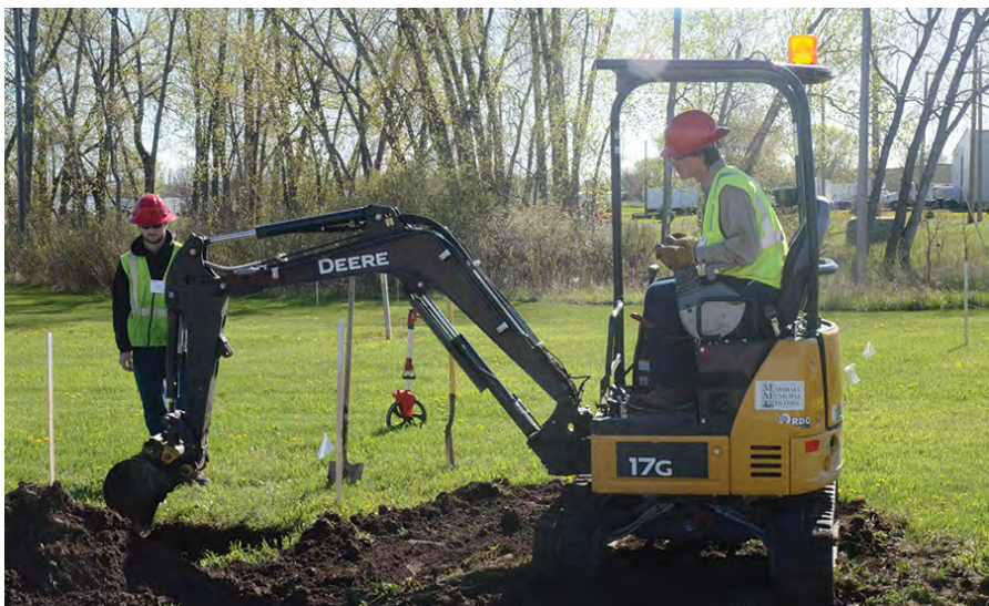
Participants practiced performing switch replacements.
