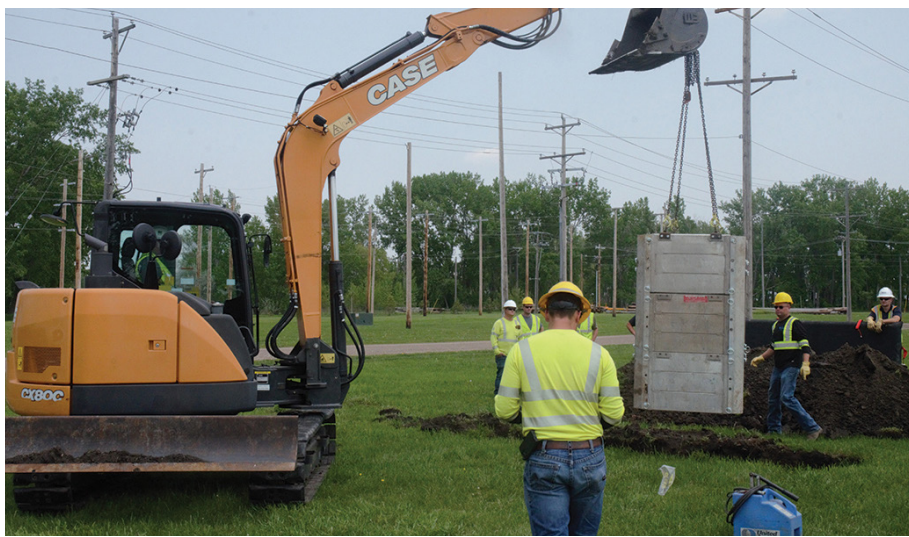
A trench box is set into the trench.
