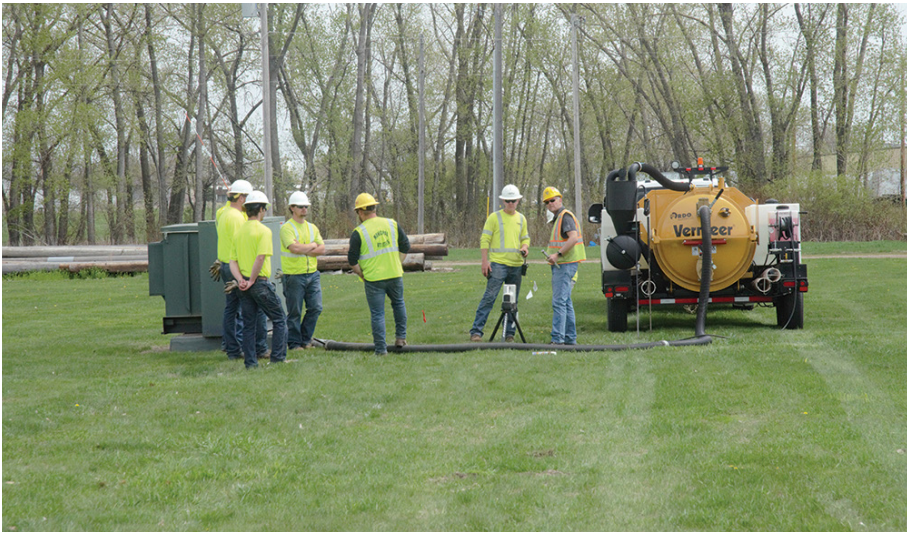
Students line up their directional drilling operation.
