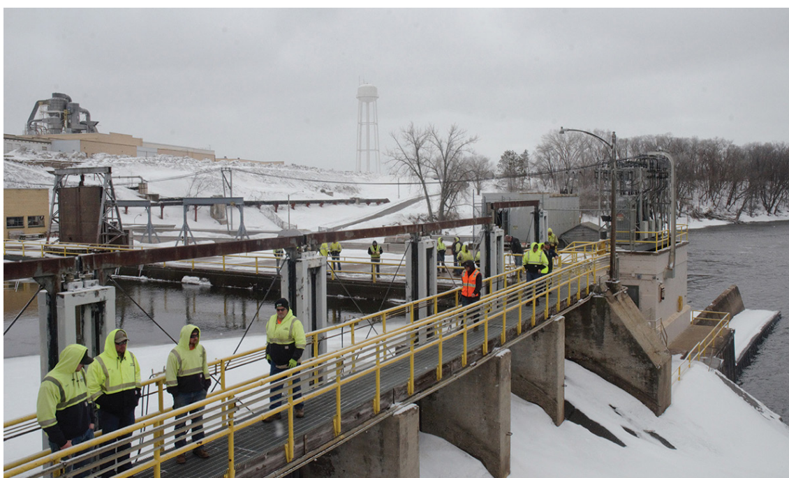
Conference attendees explored the Brainerd dam during the recent substation school.
