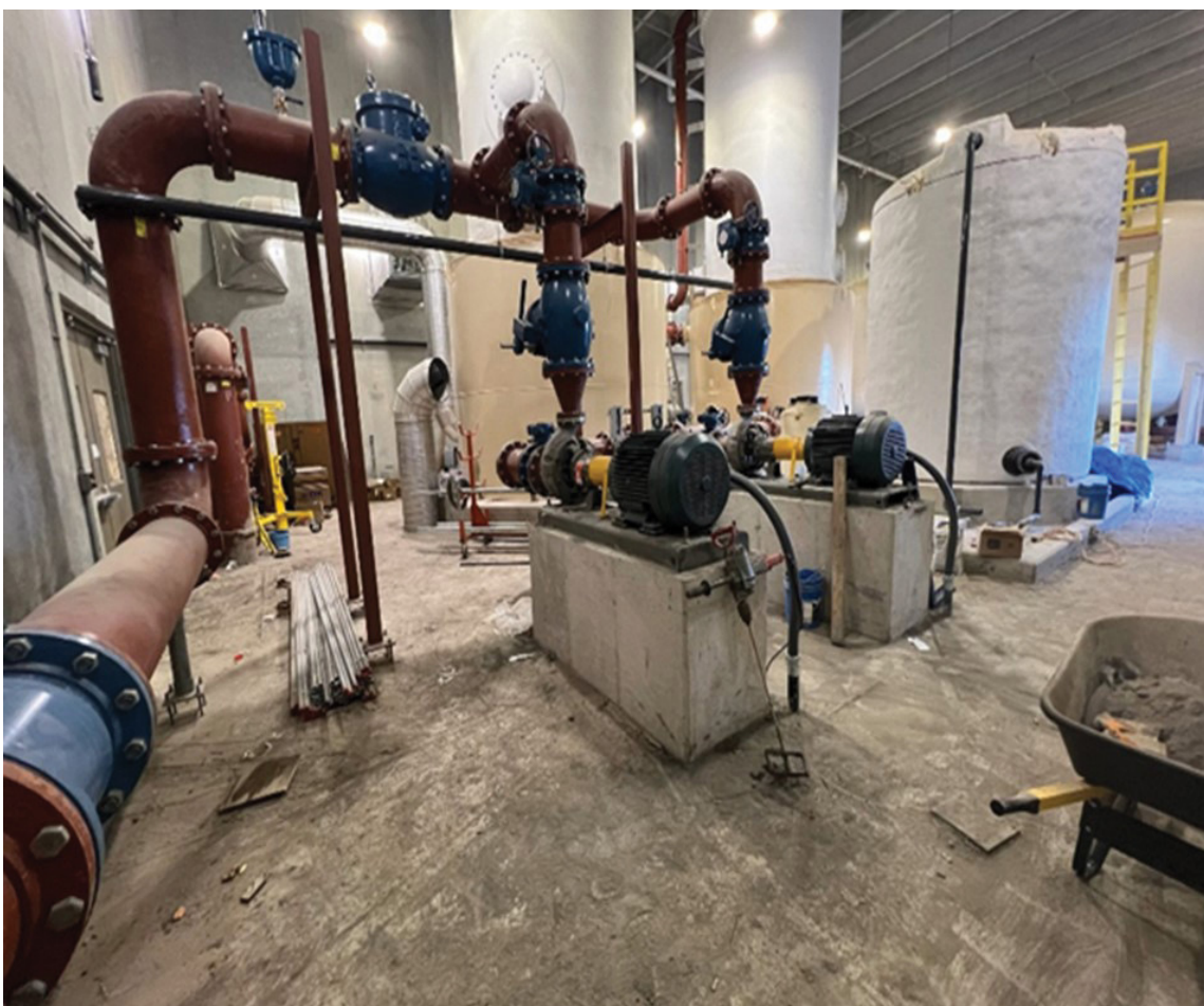
The interior of the Northeast Water Treatment Plant during construction.
