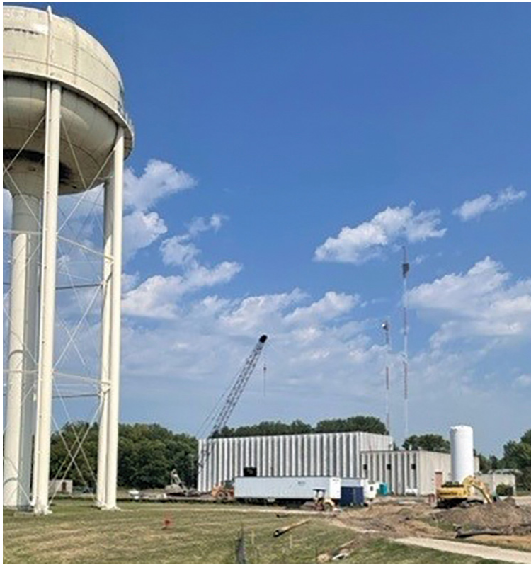
Construction is underway at the Northeast Water Treatment Plant.
