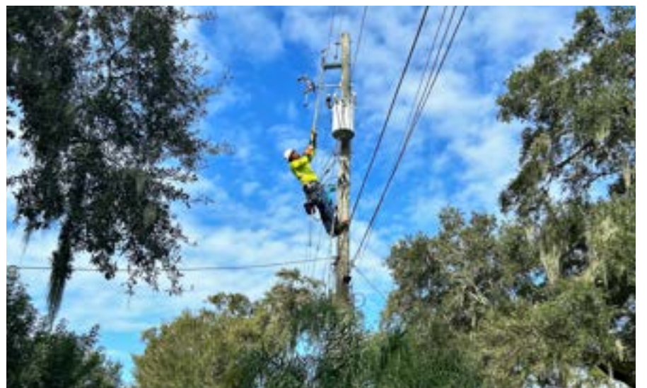
Lineworkers hook up and energize a transformer.
