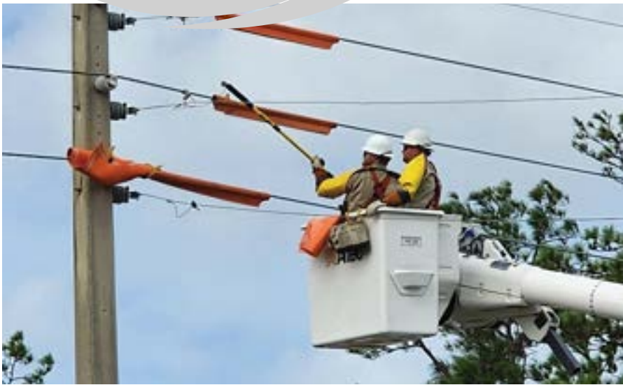
They also reenergized a span of overhead line.
