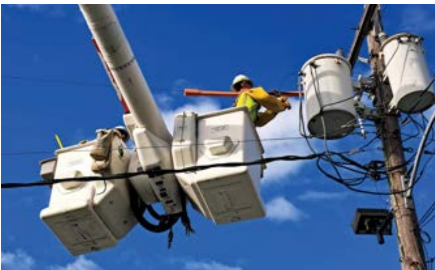
Repairing an overhead transformer bank.
