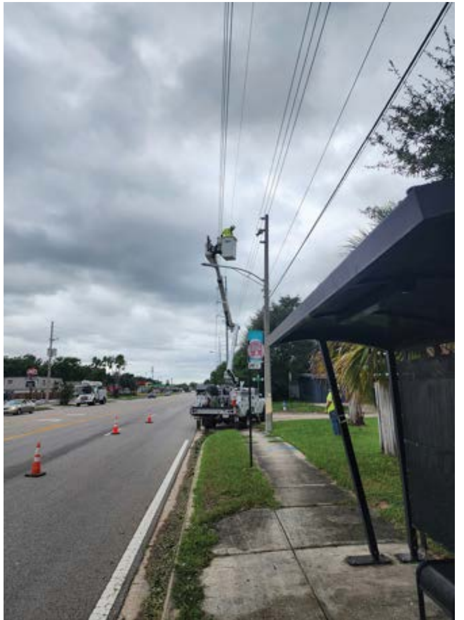
Replacing a broken tie wire on a phase.
