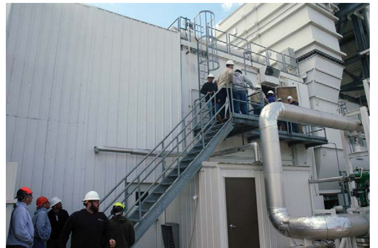
Attendees view the power infrastructure at Faribault Energy Park.
