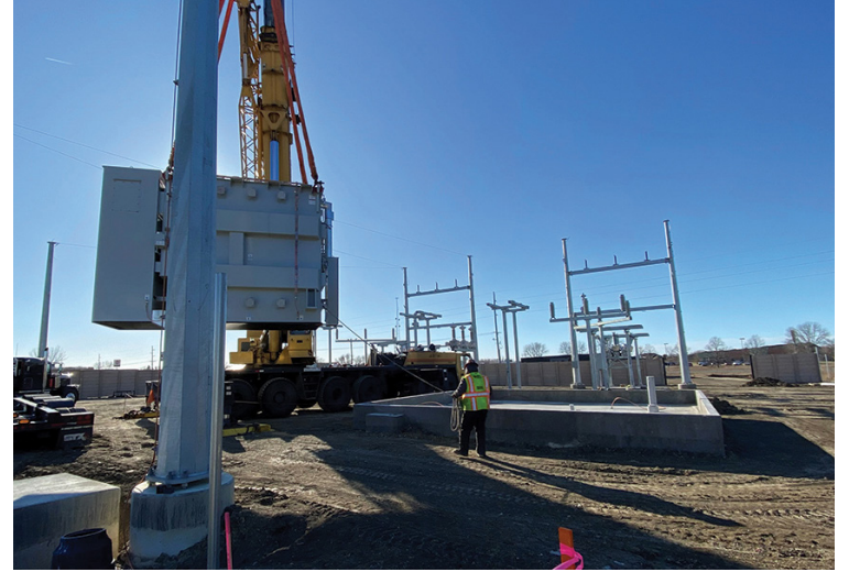
The new substation transformer being delivered and placed on December 18.
