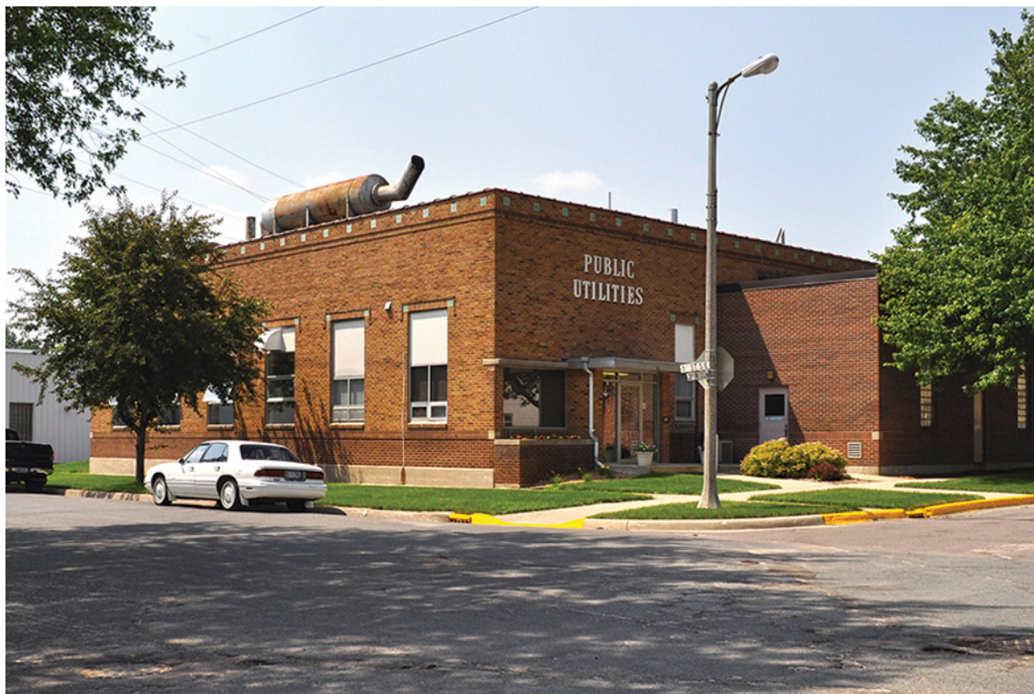
Blooming Prairie’s main public utilities building (1930) houses the #2 generator for BPPU.
