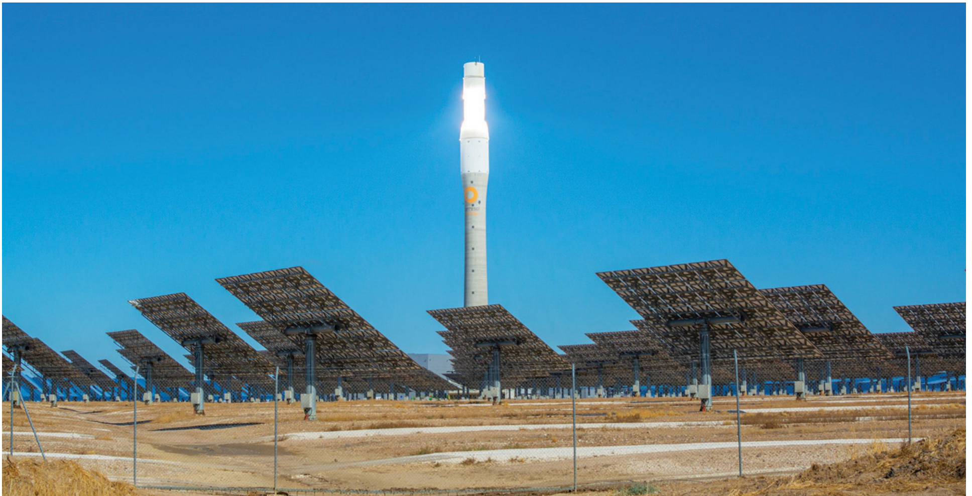
The Gemasolar Thermosolar Plant in Fuentos de Andalucia, Spain, is of the solar power tower
