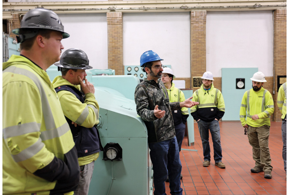
The school included a field visit to the New Ulm Public Utilities Power Plant, where Glem Hillesheim, Chief Engineer, guided participants through the facility's 6-megawatt (MW) and 15-MW generators. The cogeneration units produce electricity while supplying high- and low-pressure steam to district energy customers. Participants also toured the 3M plant in New Ulm to see how field equipment is manufactured. No photos were permitted inside the facility.
