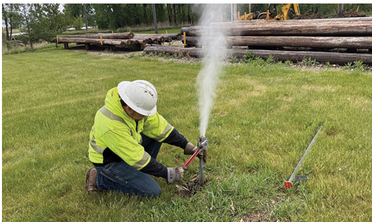
Joe Bellomy, Owatonna Public Utilities, blowing out the gas line to remove water buildup caused by inactivity.
