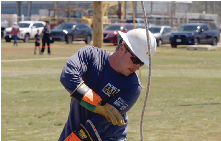
Apprentice lineworker Landon Meier from Rochester Public Utilities in action during the 2026 APPA Lineworkers Rodeo in Huntsville, Alabama.
