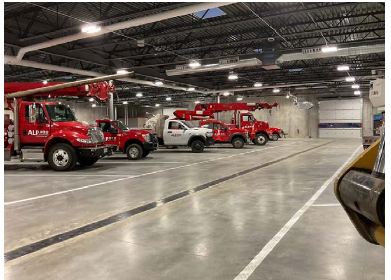
Alexandria Public Utilities' new building includes a custom garage fit to store all utility trucks perfectly.
